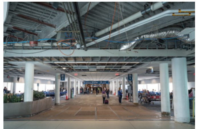
Concourse B Renovations
