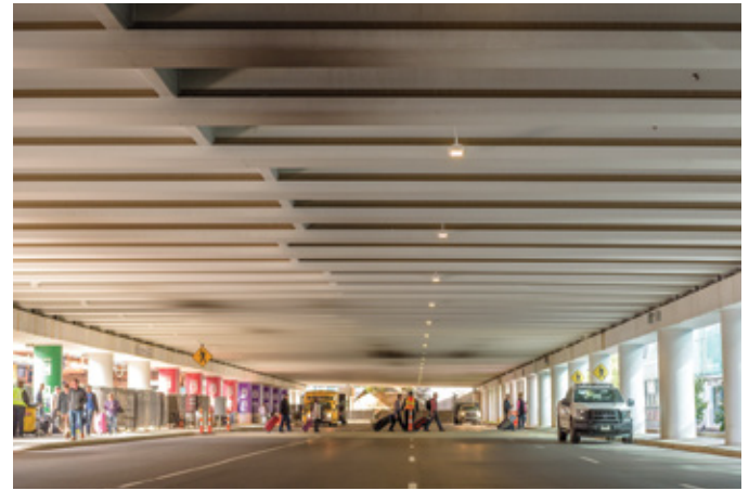
Elevated Roadway and Terminal Curb Front
